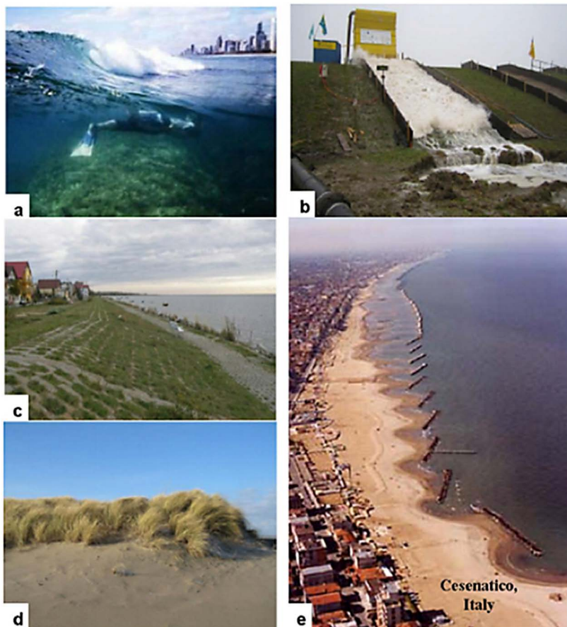
Figure 5: Technical Research and Applications on Coastal Defenses. a) submerged reefs, b) coastal dikes and simulation, c) vegetated coastal revetment, d) sand dunes stabilization, e) offshore detached breakwaters with beach preservation.
