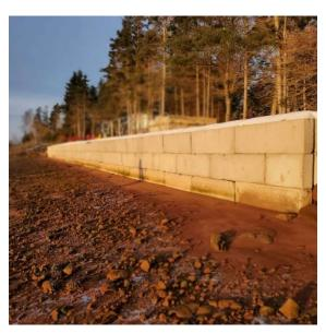
waves, he sought to deflect them in a much more aggressive way. The vertical sea wall does not absorb the force of the waves but diverts them both under and around it. As seen in the photo, it is only a matter of time before the ocean will erode under the wall resulting in its eventual collapse. Nature will always win.
