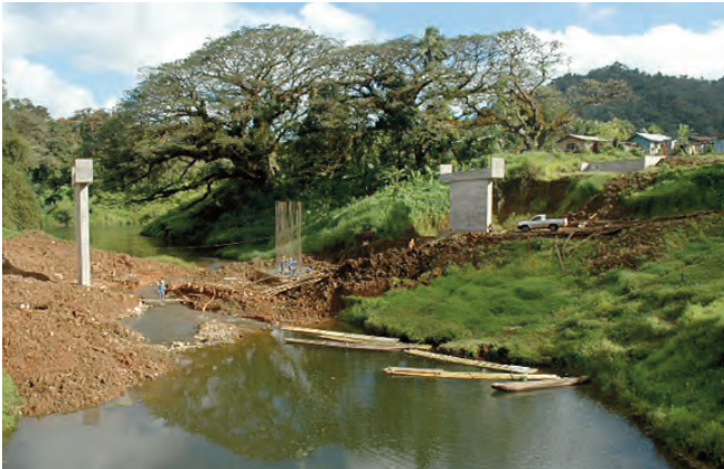
Bridge and highway construction in rural Fiji
