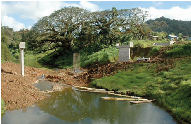
Bridge and highway construction in rural Fiji
